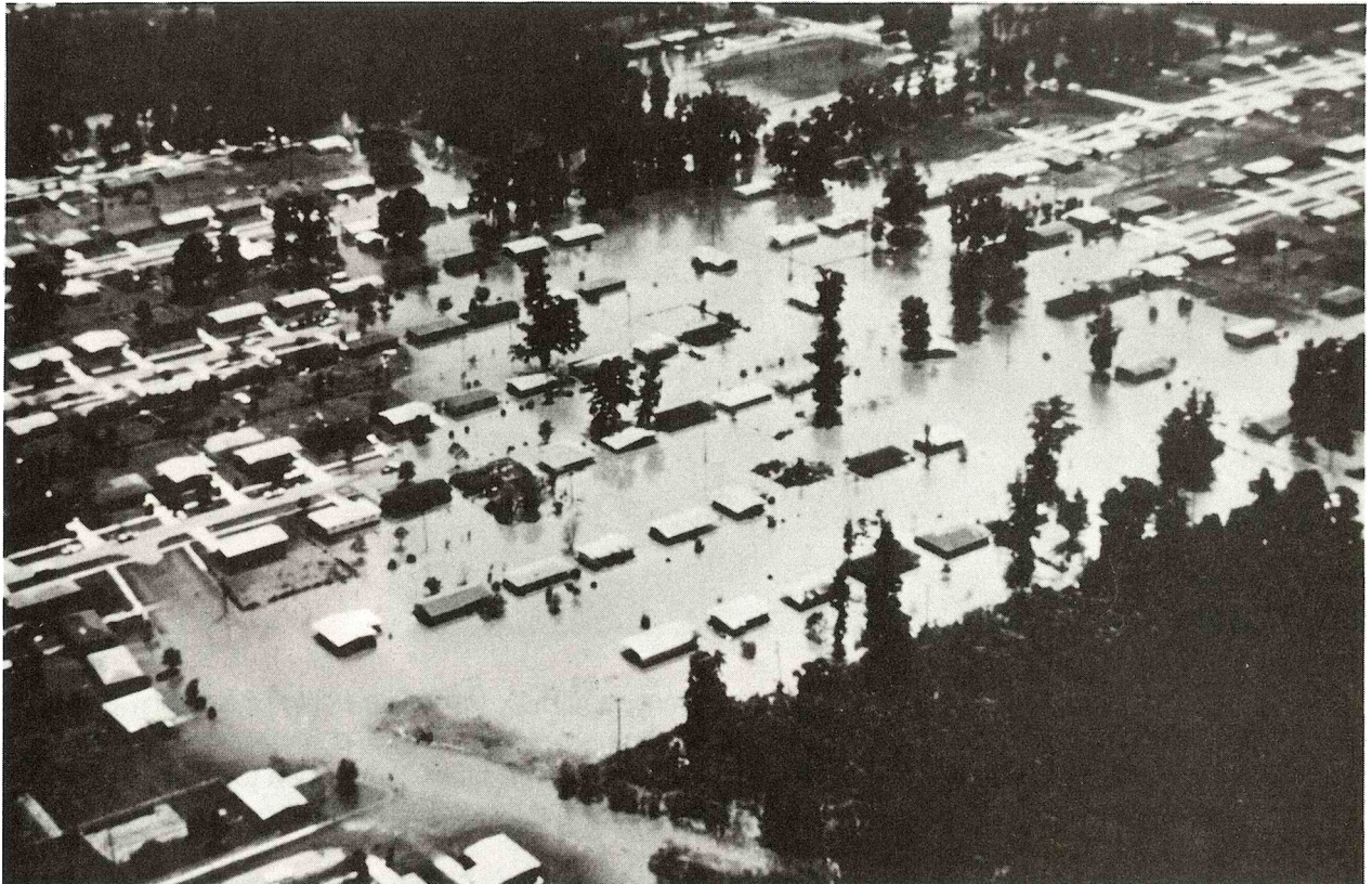
FIGURE 1-1. Flooding strikes thousands of homes every year.
