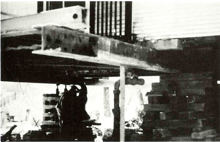
. . . while the jacks were reset to continue the lifting process.
