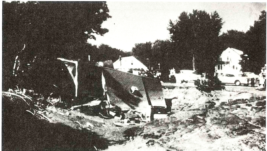
FIGURE 2-5. Erosion of the supporting soil resulted in the collapse of this house.
