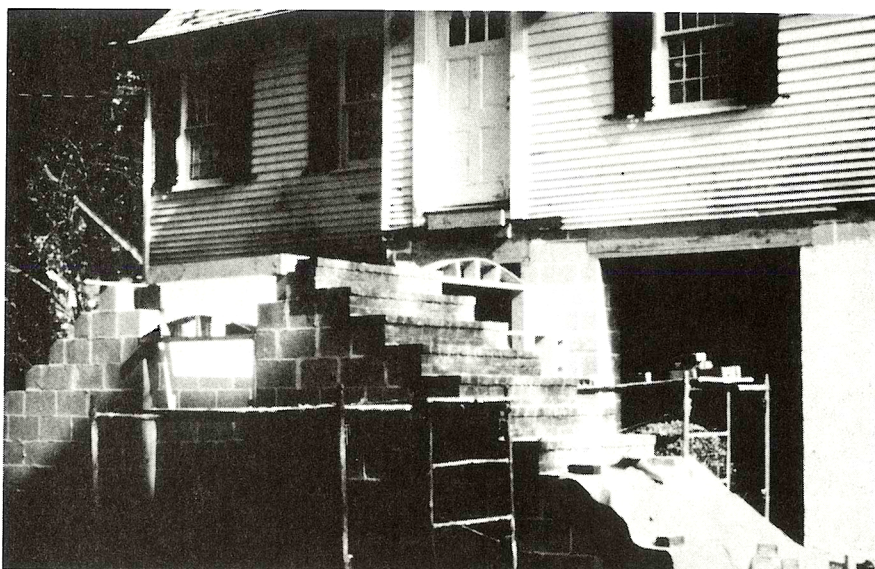
Access stairway under construction.
