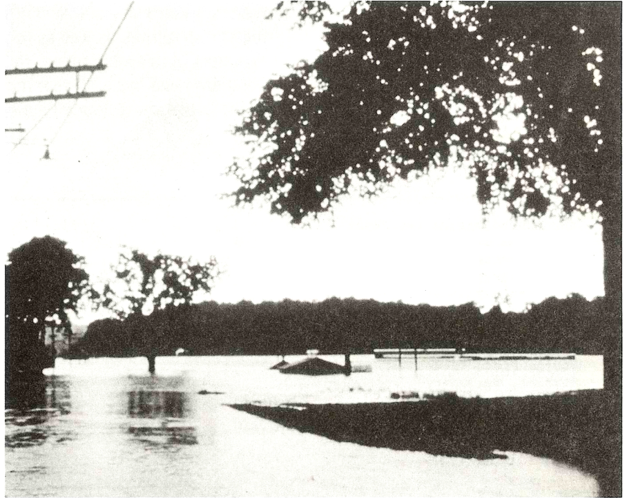
FIGURE 2-3. Deep flooding can damage or destroy any type of home.
