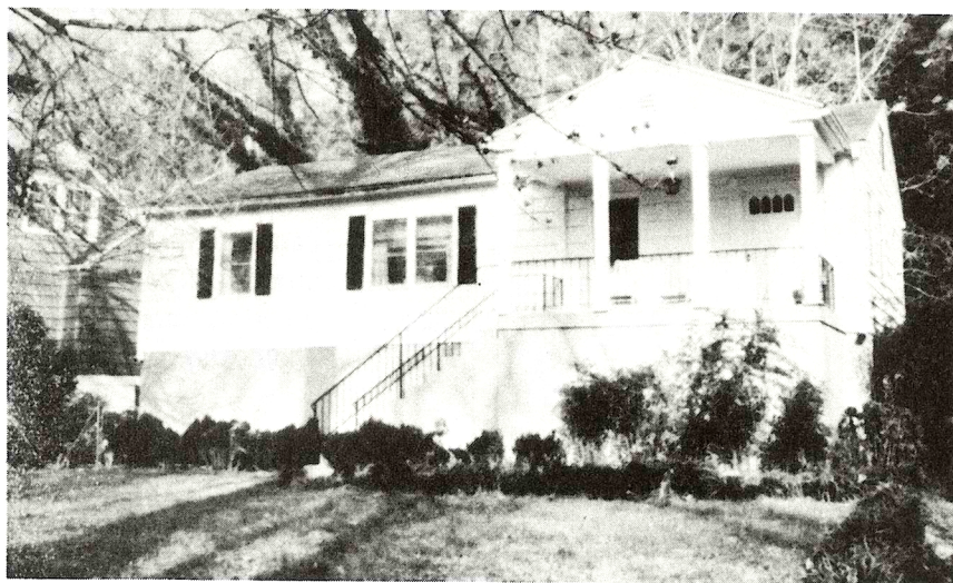
FIGURE 3-23. The owner of this house in Illinois elevated the structure ten block courses.
