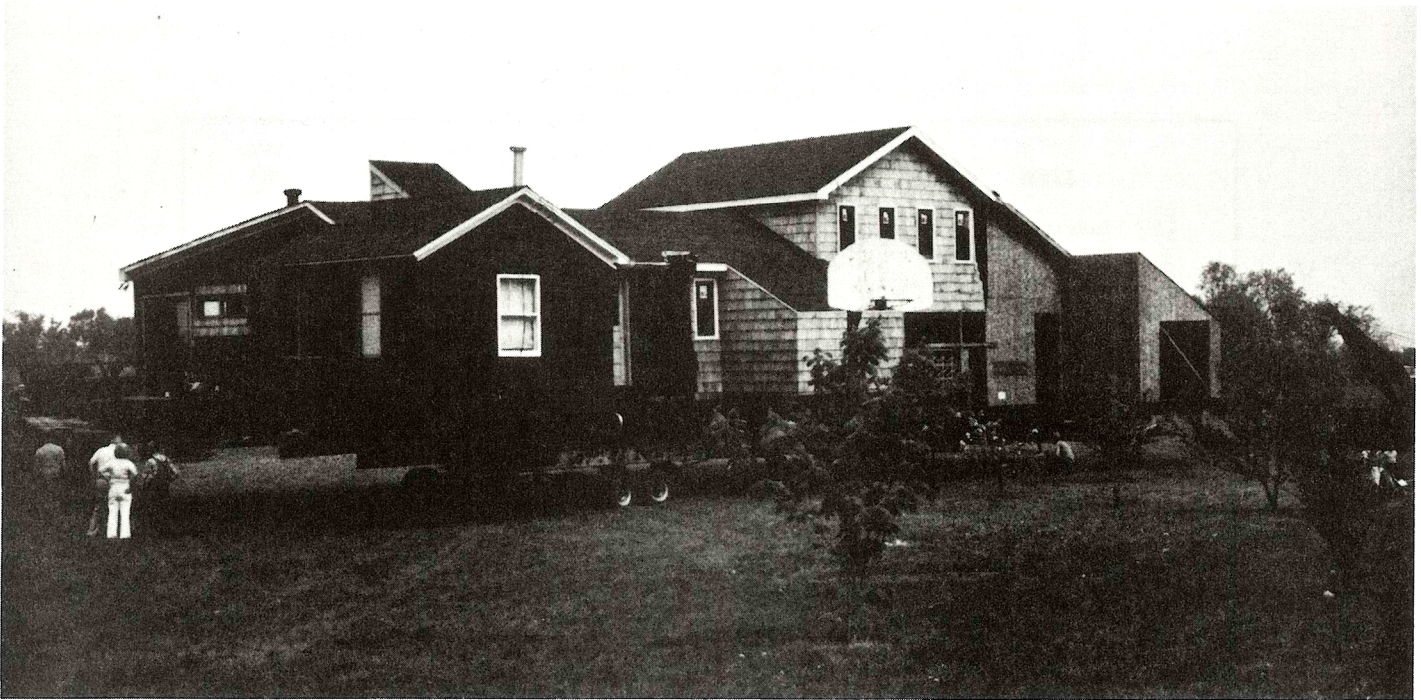
FIGURE 4-4. Even extremely large and complex structures can be successfully relocated.
