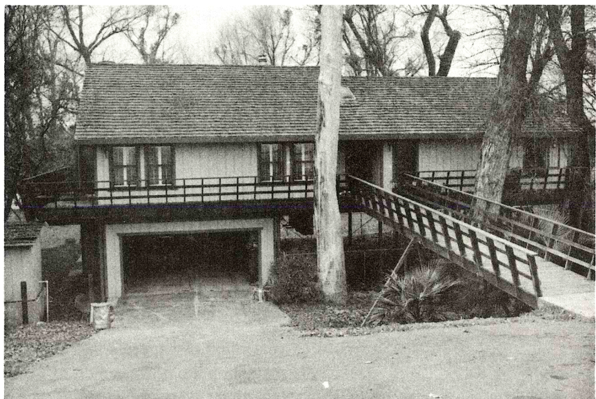
FIGURE 3-9a. A walkway to an elevated house near Sacramento, California doubles as an escape route. These photos show the house in both a flooded and unflooded condition.
