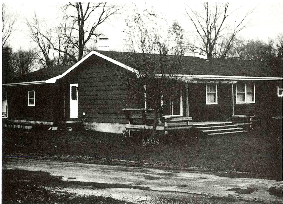
FIGURE 3-3. The owner of this house in Illinois elevated his house the height of only three masonry blocks, but in this case, it significantly reduced the exposure to flood damage.
