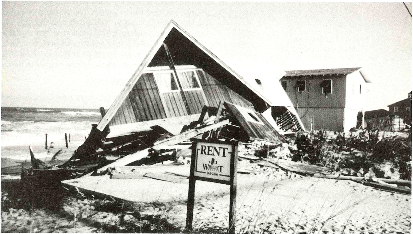
FIGURE 2-2. Because of velocity wave action and high winds, flood damage is more severe in coastal areas.
