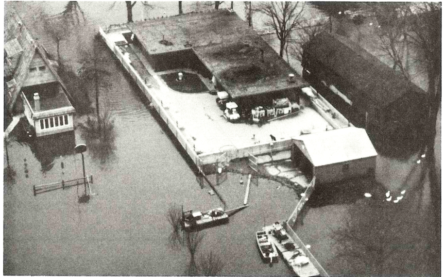
FIGURE 6-5a. In times of flooding, floodwalls act to keep water completely away from the structure.
