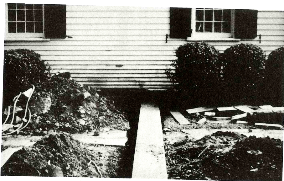
Lifting beams were then inserted . . .
