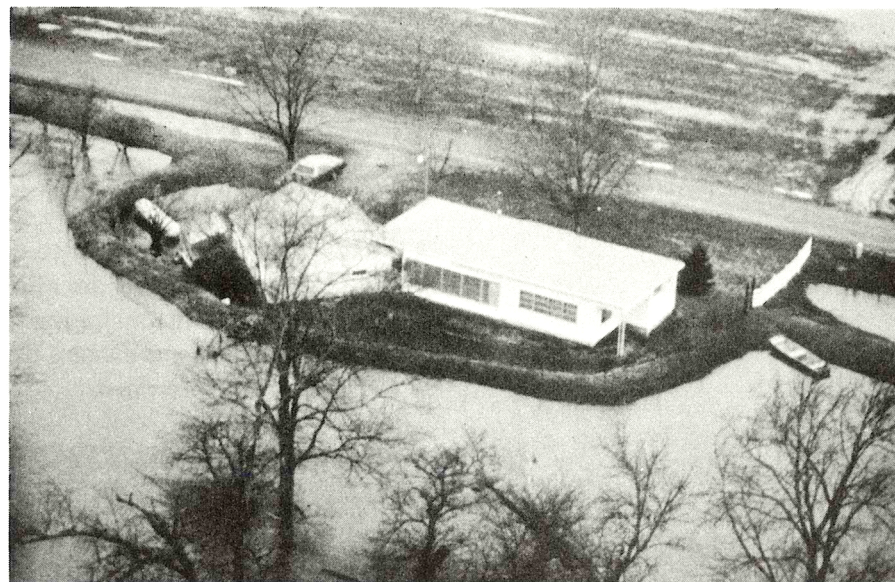
FIGURE 5-3. By using a levee as a retrofitting technique, a homeowner may not have to alter the structure in any way.
