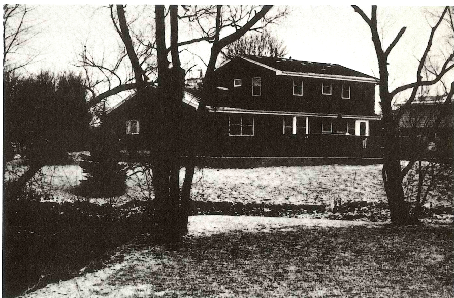
FIGURE 1-9. The floodwalls are both attractive and effective flood protection.
